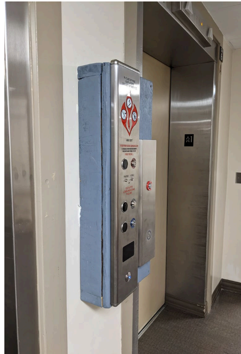
Non-code compliant elevator hall station
