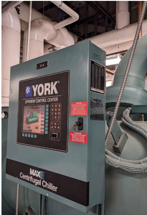
Control panel from an illegally installed chiller
