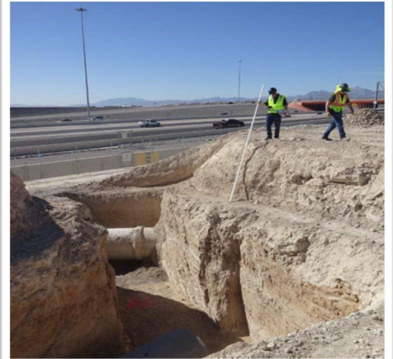
Supervisor and CSHO measure a trench.
